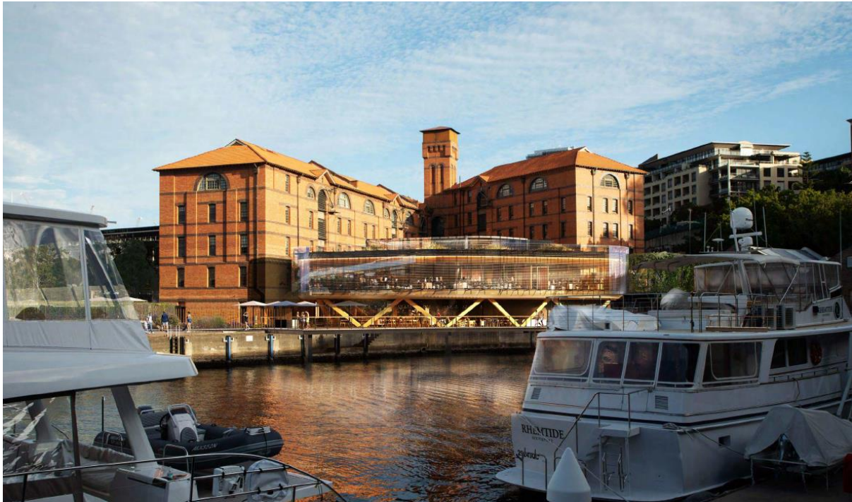
Figure 40: Photomontage looking east across to the subject site from Jones Bay Wharf
