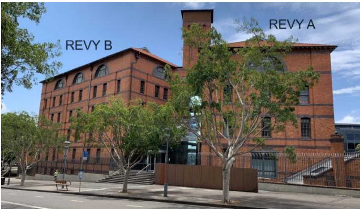
Figure 6: Pirrama Road elevation, noting principal building entrance is currently provided along this frontage
